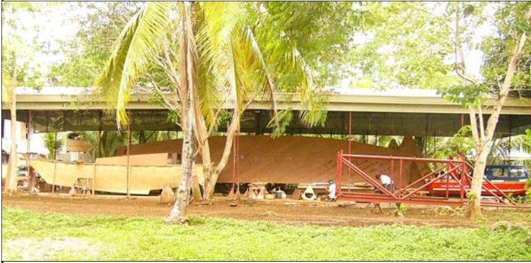
Andy Smith's yard with Islander 65 under construction
